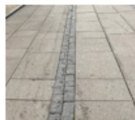
Fig. 110: Tactile guide line being used in the pedestrian path, section view, 20 cm width (Landscape)
