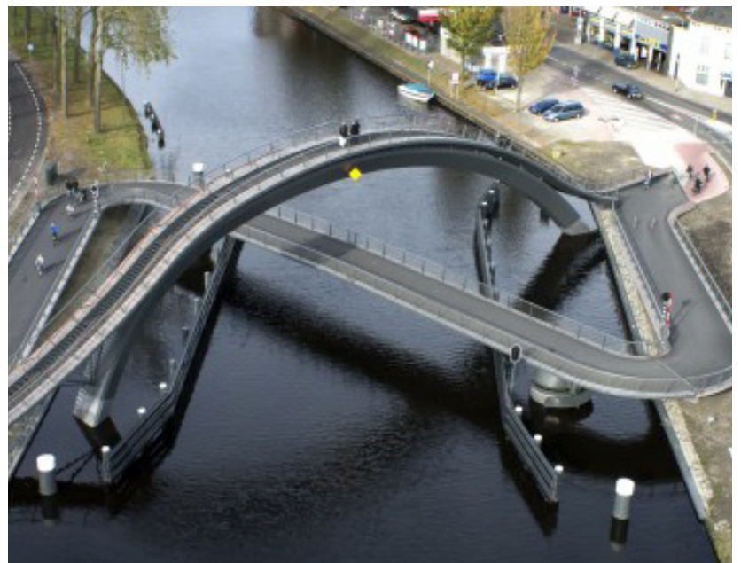
Next architects, Amsterdam
